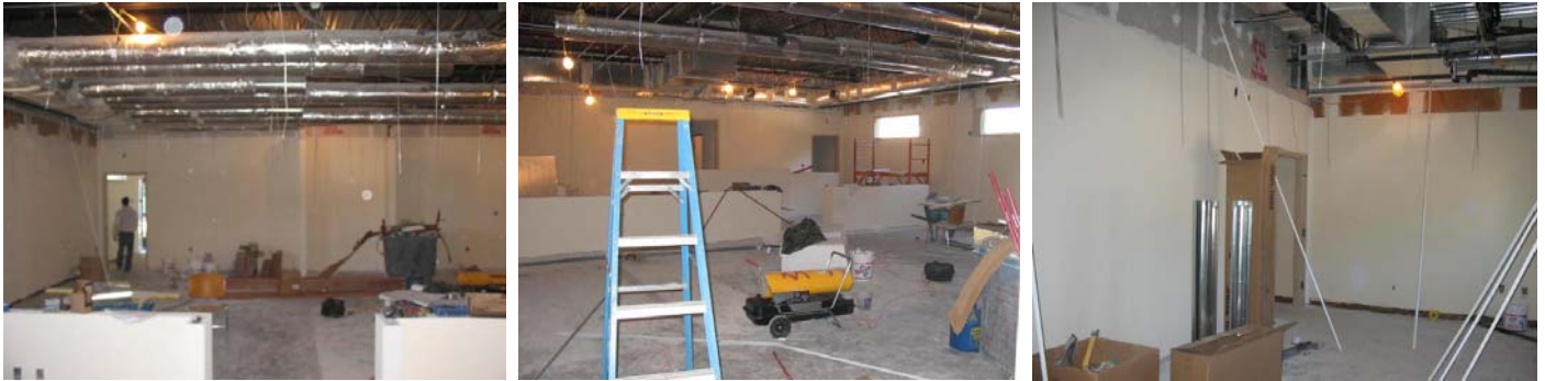
Courtroom During Construction
